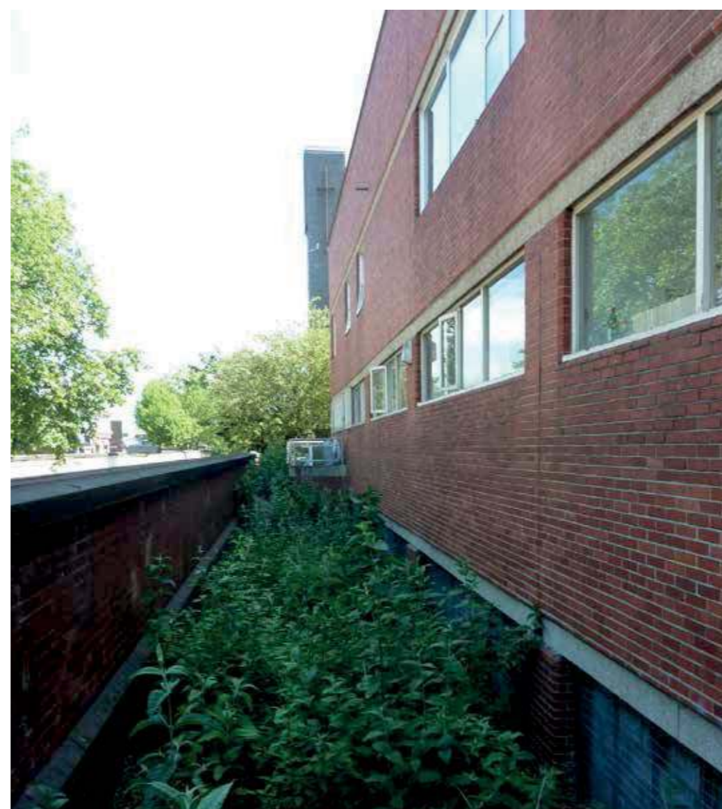
View D: Rear of the Civic Centre next to the Rotherhithe Tunnel a
